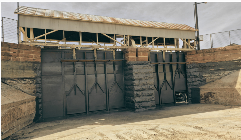
Photo courtesy of J.Conrad (main headgates)
